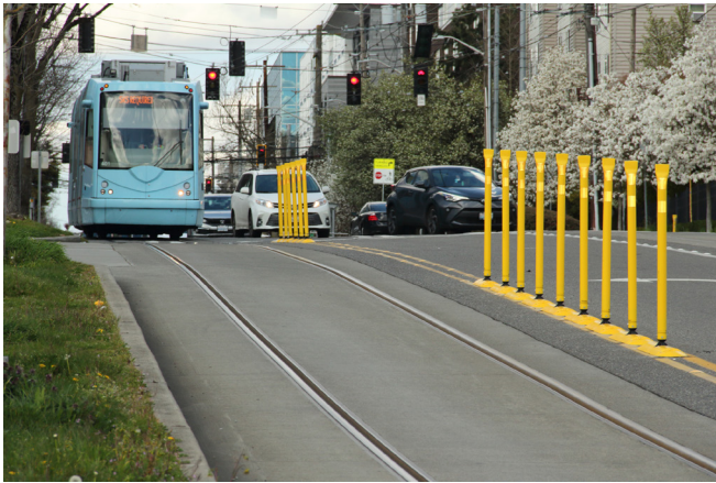
Broadway and Alder tuff posts
